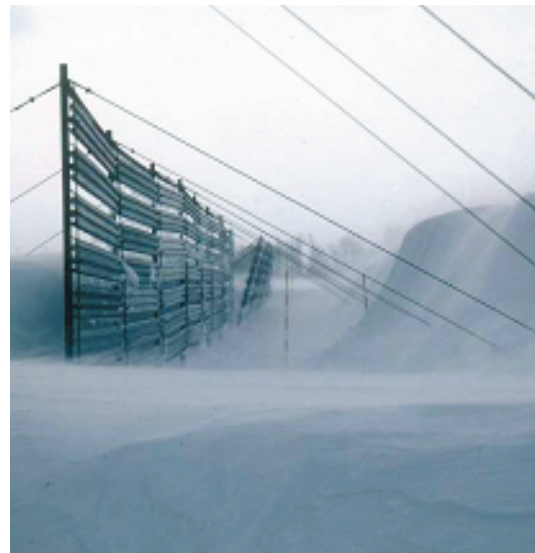
▲吹きだめ式防雪柵
