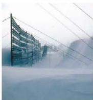
▲吹きだめ式防雪柵
